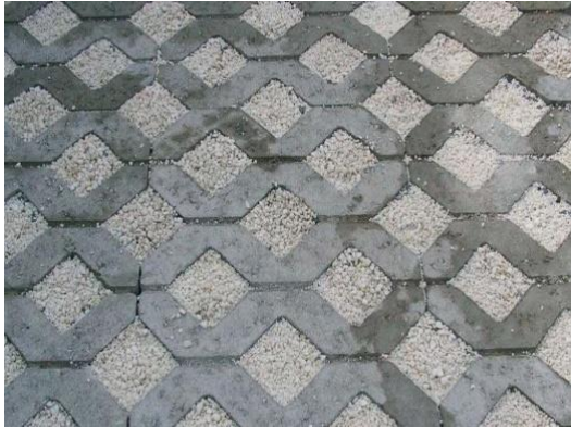
Plate 4-32 Example of filter drains and permeable surfaces
